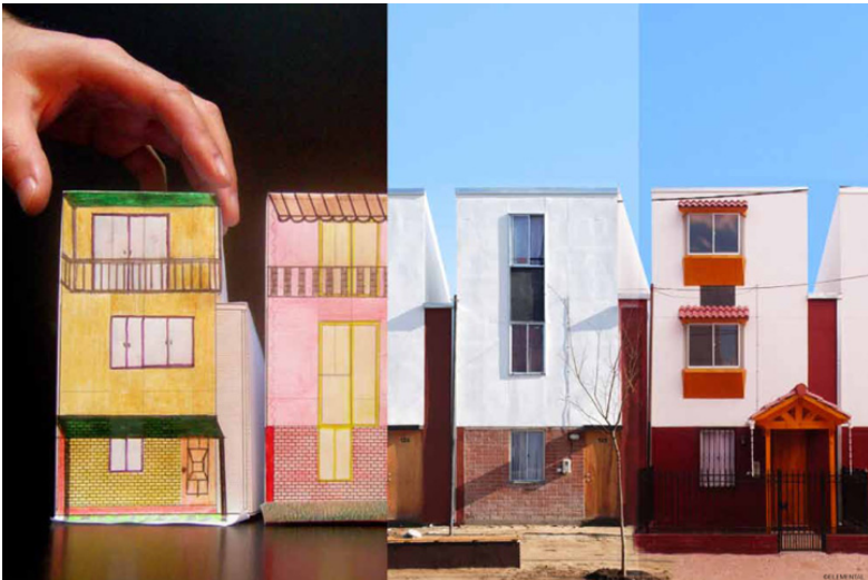
Fig. 2 Collage depicting three stages of development. Left: models used in a co-design session with future residents. Middle: completed construction. Right: after being lived in for some time, showing modifications by the residents. Source: Elemental
