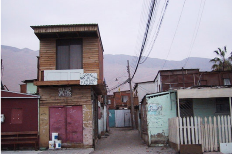
Fig. 1 Quinta Monroy, as seen here before Elemental's project, is representative of Chile's informal urban settlements. Source: Elemental
